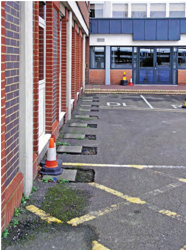
Ground sockets in front of the windows of part of the council offices at Dartford. These were explained by a former official as having been for the insertion of timbers to be faced by thick planking, against which a bank of sand was to be piled to give protection to the ground-level control centre behind
